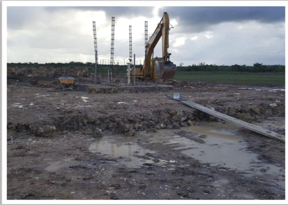
Cisco's Heavy Equipment utilized for setting up foundation for Tower #4
