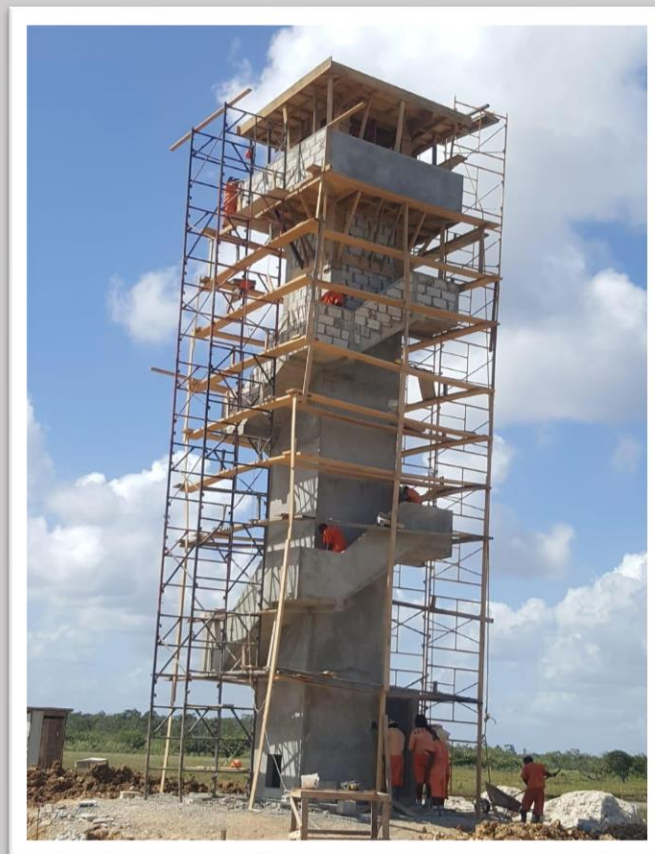
Construction of Tower #4
