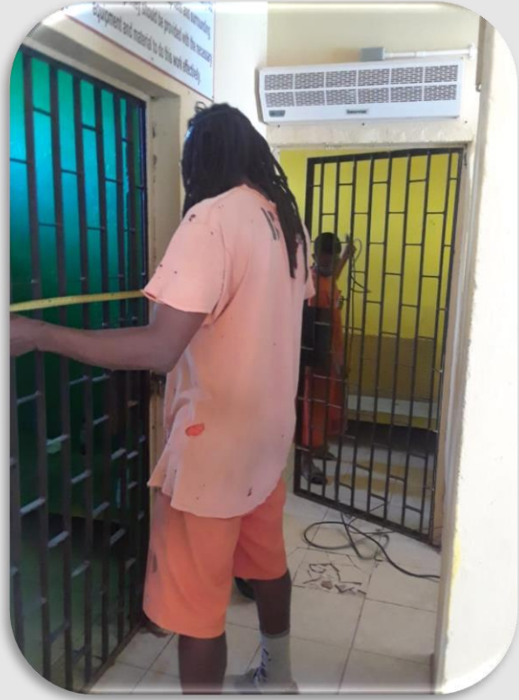
Welding repairs to wickets
