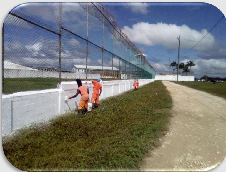
White liming of outer perimeter fence base by inmates
