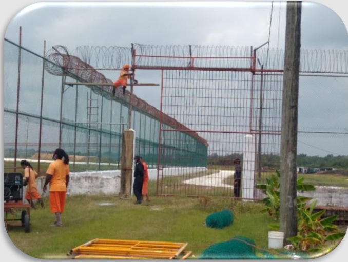
Repairs to outer perimeter fence
