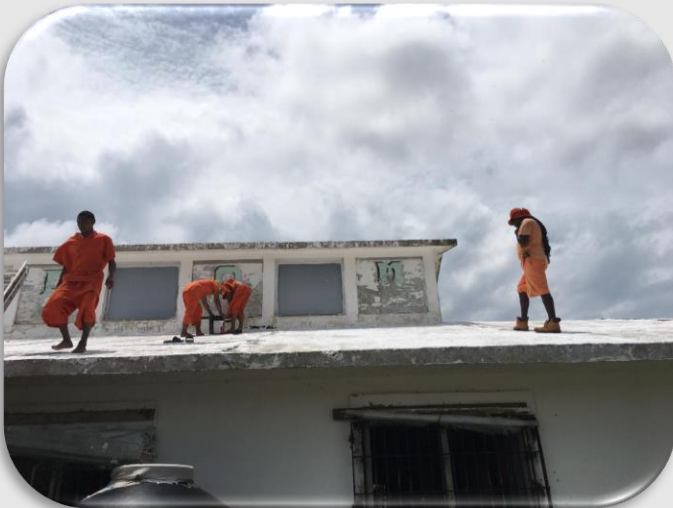
Scraping and Painting of the Tango 1 Building
