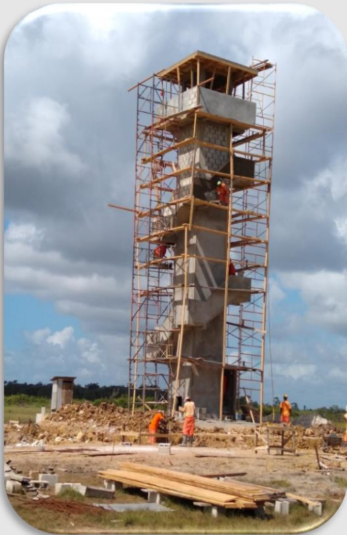
Construction of Tower #4
