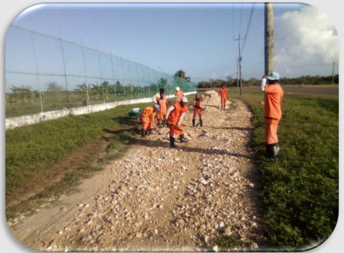
Outer perimeter road maintenance
